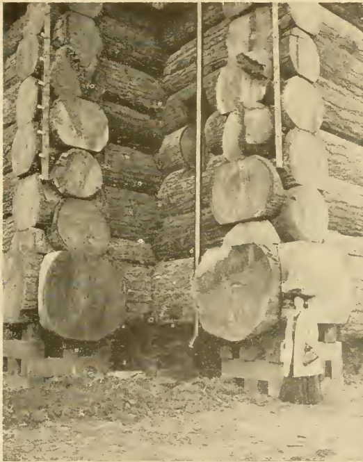
A CORNER OF THE FORESTRY BUILDING
